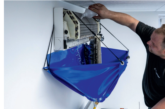
Clean split indoor units on site with the Foldable Funnel
